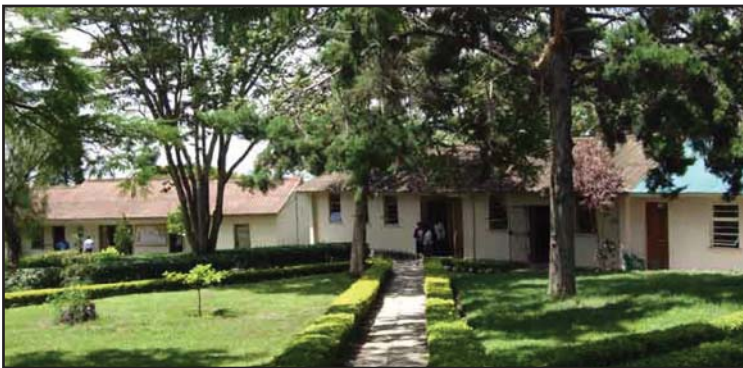
Classroom buildings at Mount Meru University in Arusha, Tanzania.
